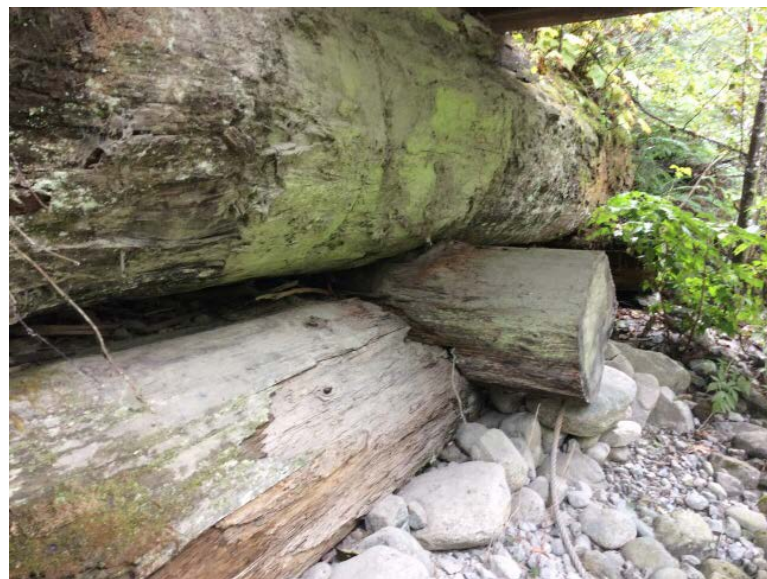
Left Bank Abutment when facing downstream
