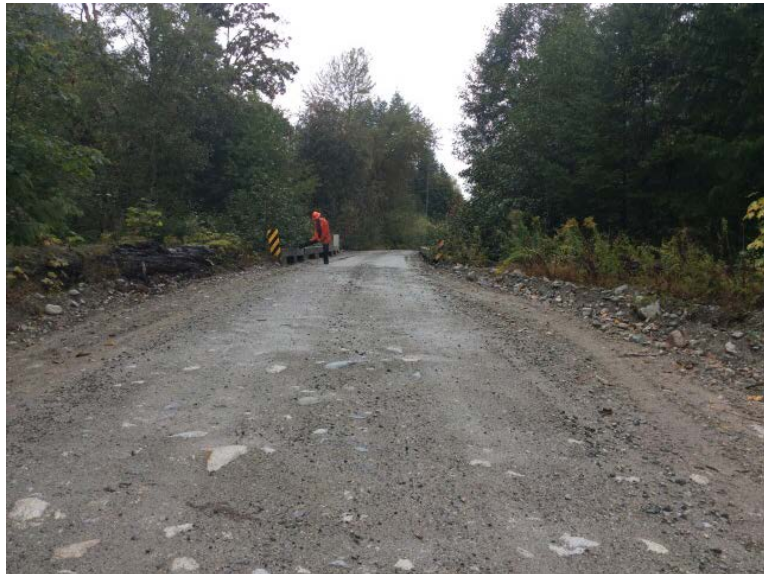
Approach from Right Bank when facing downstream
