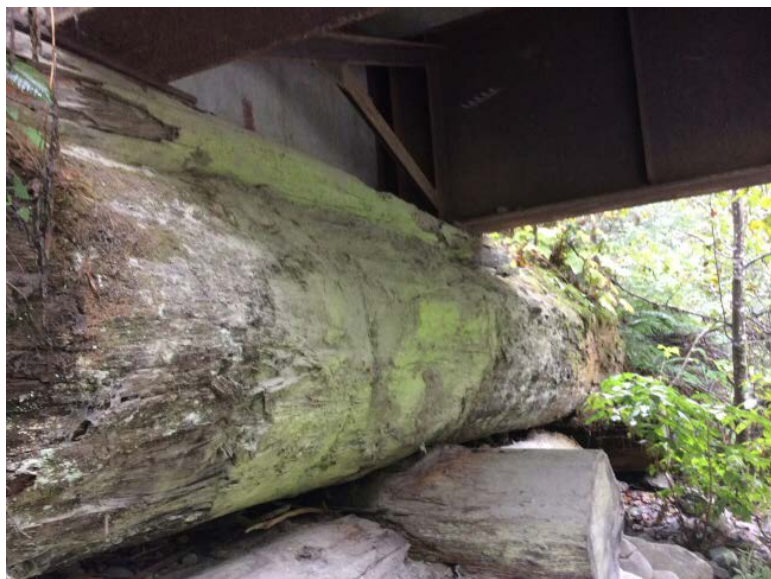
Left Bank Abutment when facing downstream
