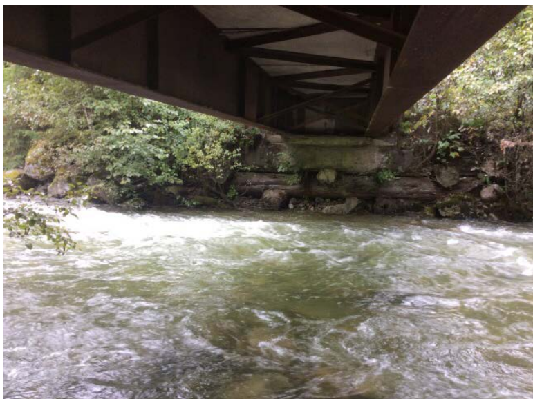
Right Bank Abutment when facing downstream
