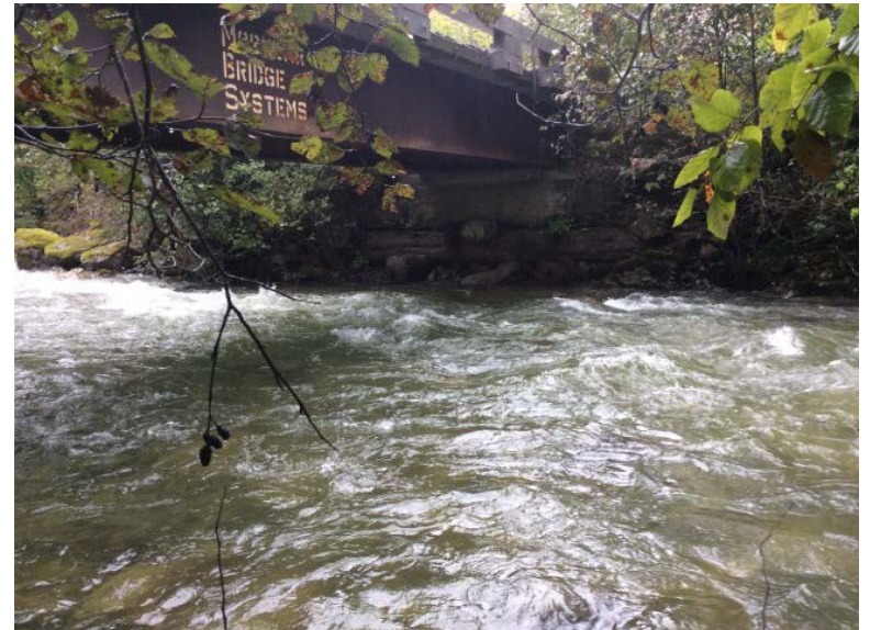
Right Bank Abutment when facing downstream
