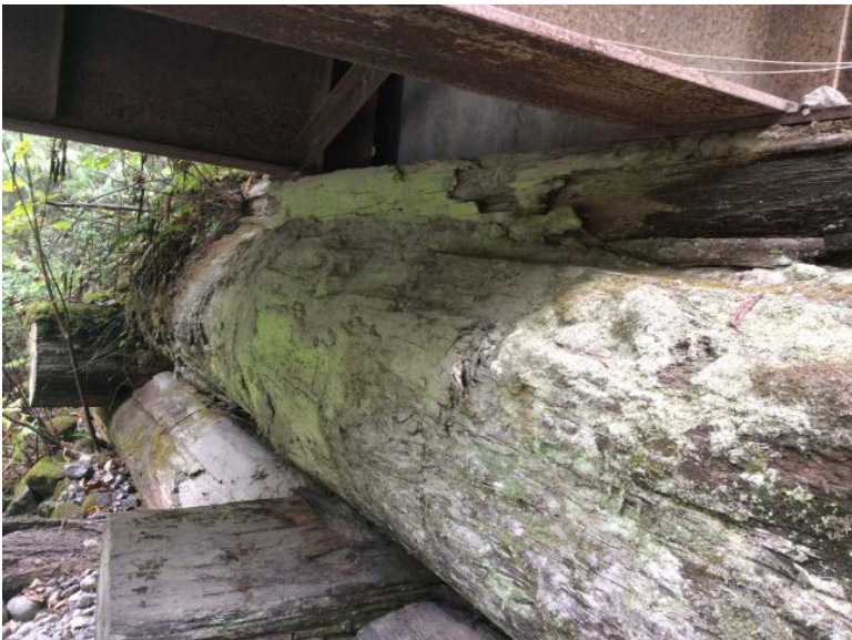
Right Bank Abutment when facing downstream
